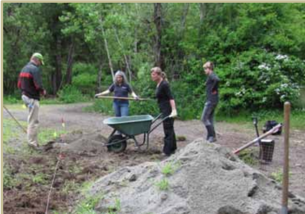
Many wheelbarrow loads of sand and soil were moved to provide sufficient depth (20 cm or more) to the nesting areas.
