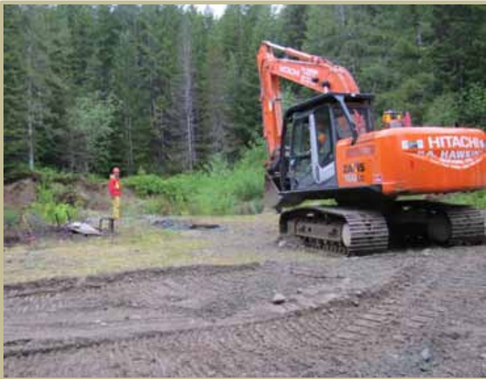
Heavy machinery arrived to prepare the ground, courtesy of Island Timberlands.
