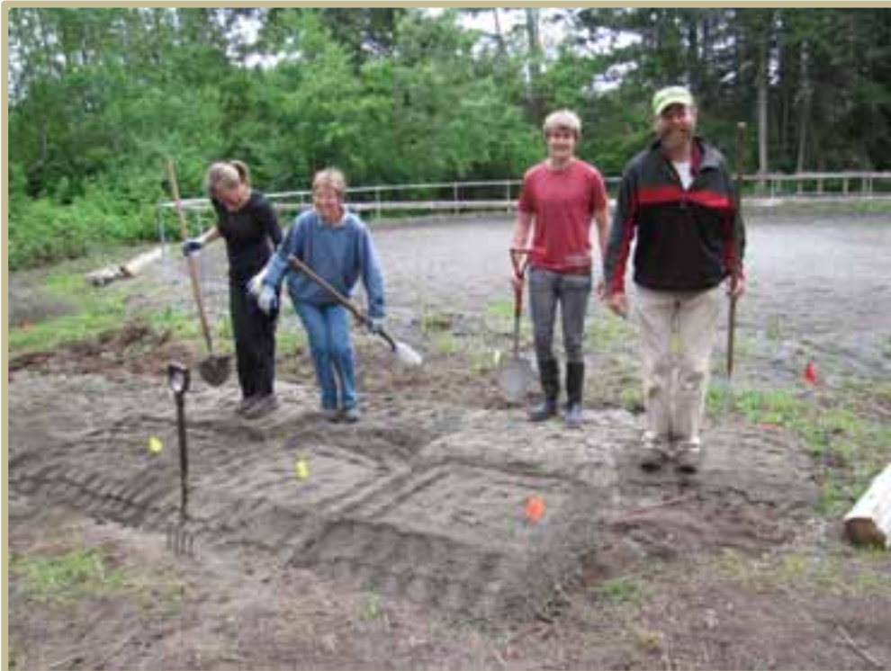
Compacting the substrate.
