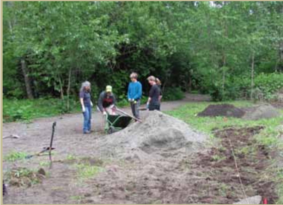
First, the ground was cleared of weeds, and piles of sand and soil were brought in, courtesy of CRD Parks. EBES donated a pile of sand already present at the site.
