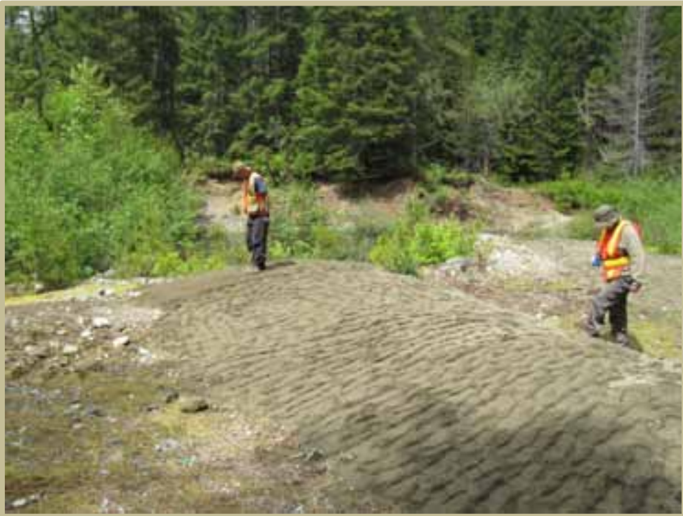
Walking on the ridges to compact the sand.
