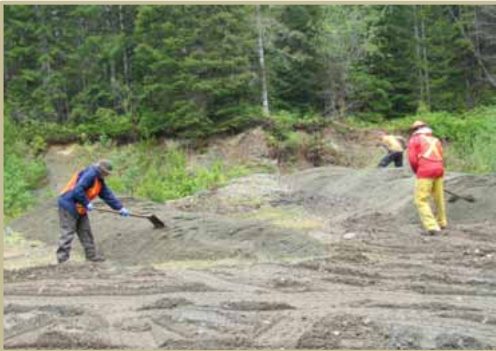
The ridges were shaped to create a gentle slope on the south-facing side.
