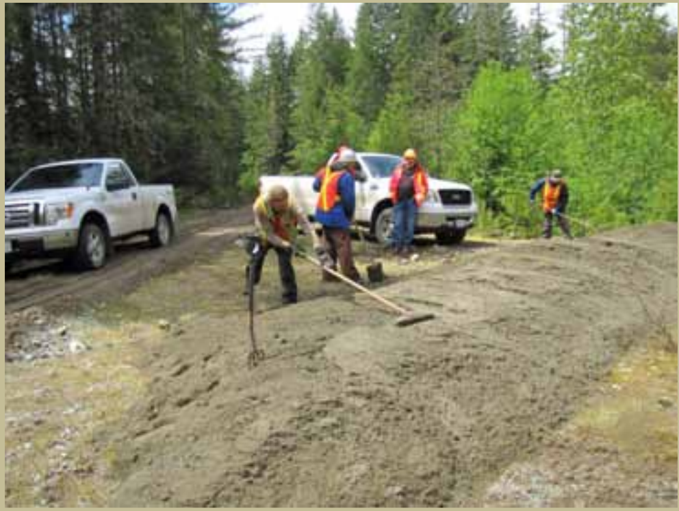
Raking the slope; Island Timberlands personnel inspecting the work.
