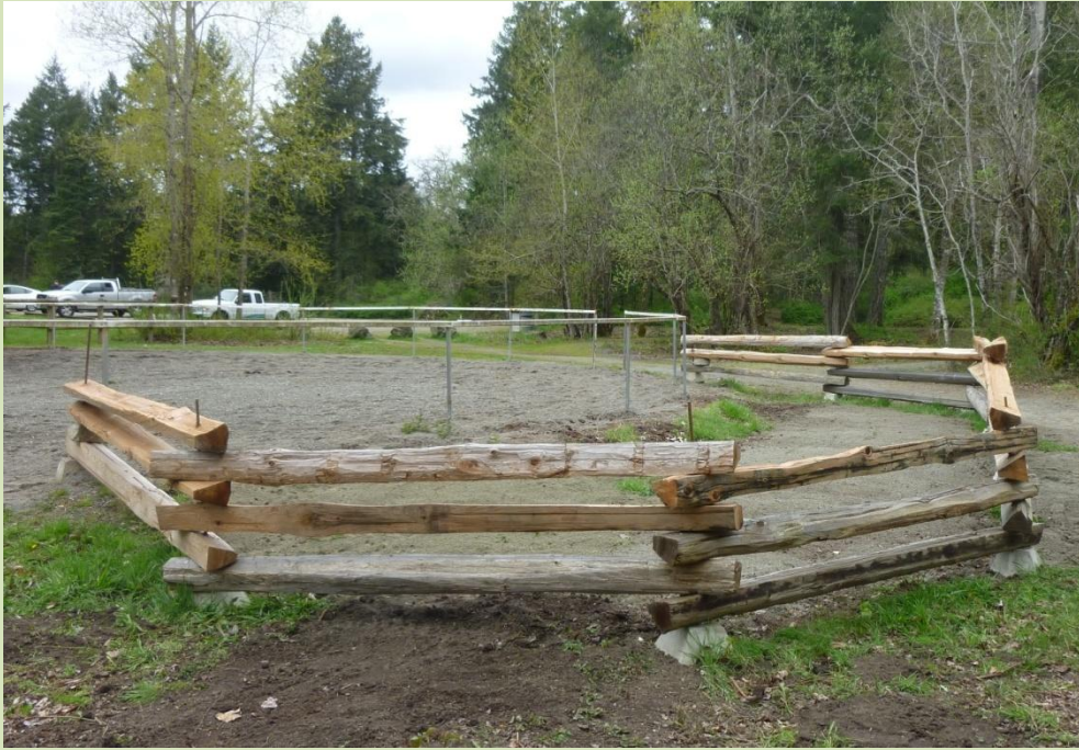
An additional tier was added to the cedar "snake" fence to reduce disturbance.
